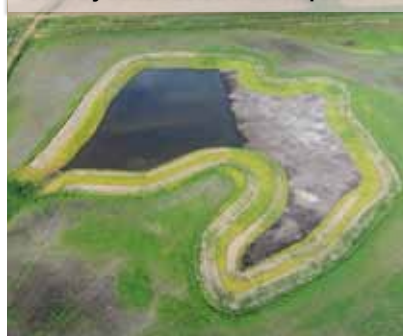
A pipe from the channel feeds a large, recently constructed habitat pool
